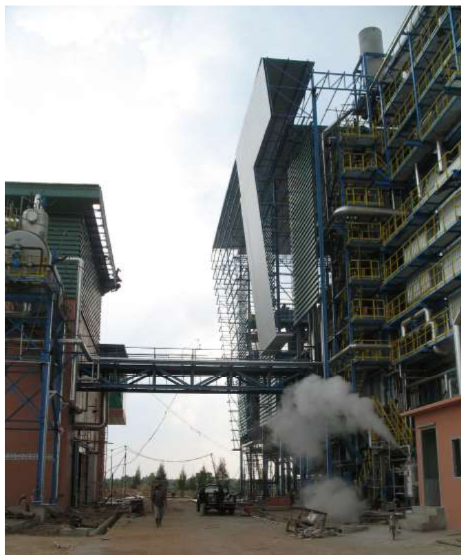
ERECTION - BOILER WITH BOILER HOUSE, WALK WAY
