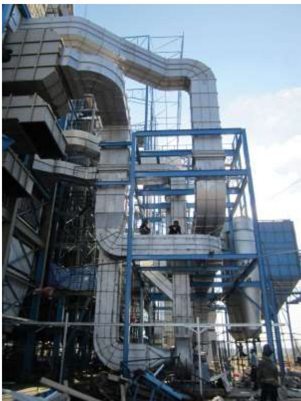
ERECTION - GAS DUCT SYSTEM, CYCLONES
