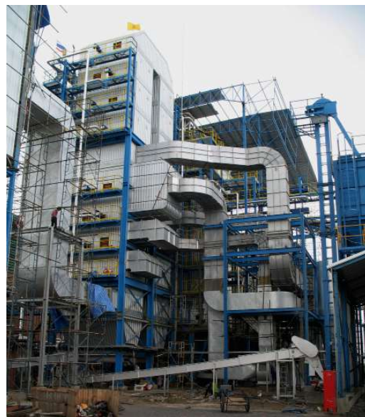
ERECTION - COMBUSTION SYSTEM - COMBUSTION CHAMBER, FUEL TOWER WITH DOSING, GAS DUCT SYSTEM
