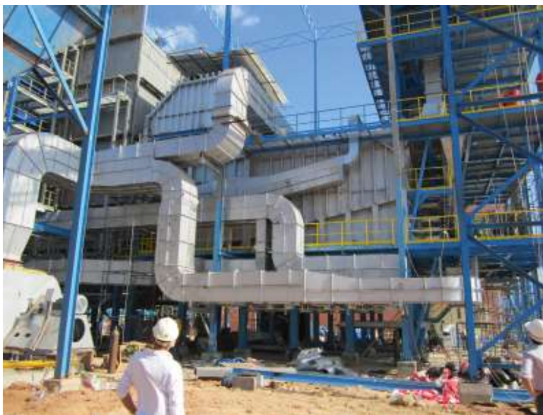
ERECTION - COMBUSTION SYSTEM - COMBUSTION CHAMBER, FUEL TOWER WITH DOSING, GAS DUCT SYSTEM
